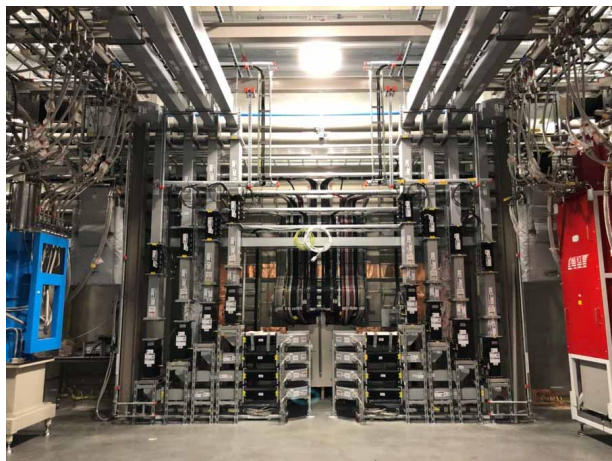
Figure 2: The cells with RFDS run between the klystrons in the RF Gallery and the cavities in the tunnel.
