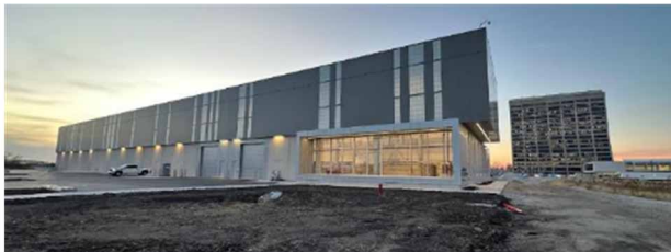
Figure 4: Cryogenic Plant Building.
