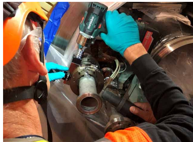
Figure 3: Cutting helium process pipes to length.
