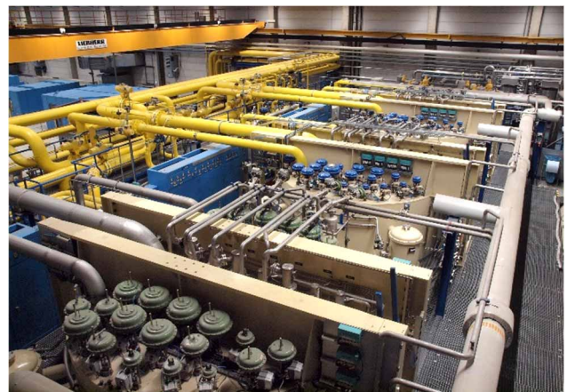
Figure 5: The cryoplant cold boxes.
