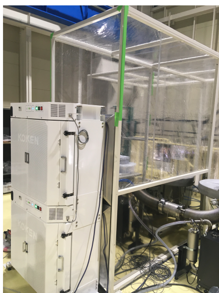
Figure 4: Newly installed clean booth.
