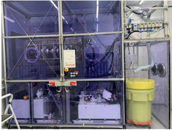
Figure 1: FRIB electropolishing facility with \beta=0.80 six-cell elliptical cavity connected to system in preparation for commissioning EP process.
