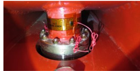
Figure 6: Heaters installed on the prototype SSR1 vacuum vessel to warm the strongback up.
