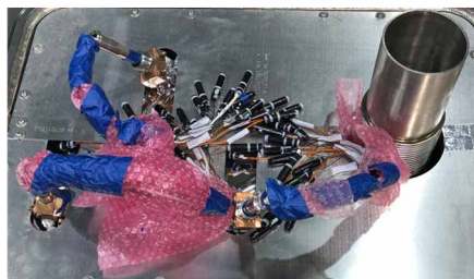
Figure 7: Wires through the pressure transducer lines.
