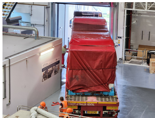
Figure 9: Trailer after delivery at STFC-UKRI. Note sharp trailer angle relative to the entry door to avoid the experimental hutch (left).
