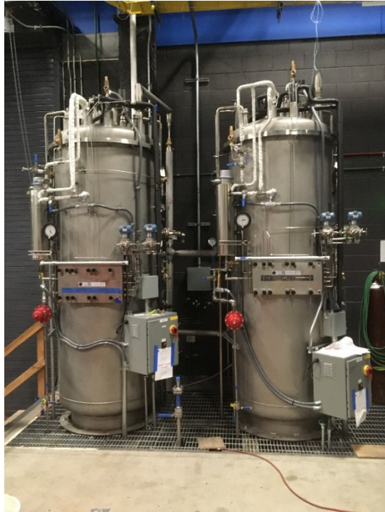
Helium purifiers (left) and compressor (right) (Located in FRIB compressor room)
