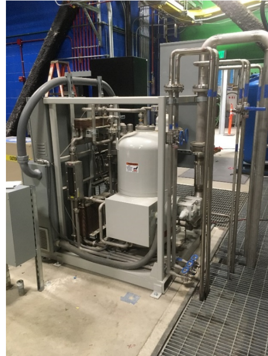
Helium purifiers (left) and compressor (right) (Located in FRIB compressor room)
