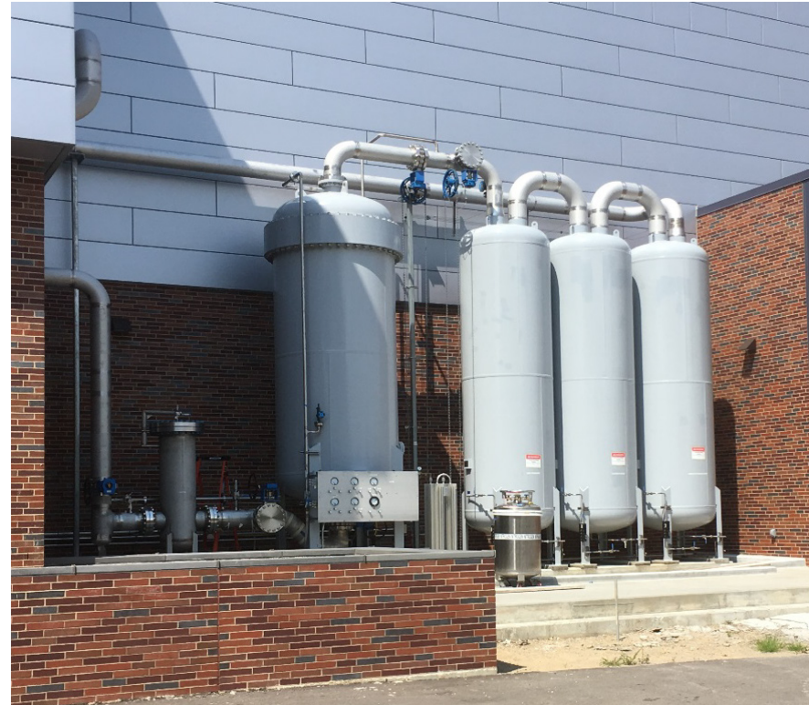
Final oil removal (outside, south side)
