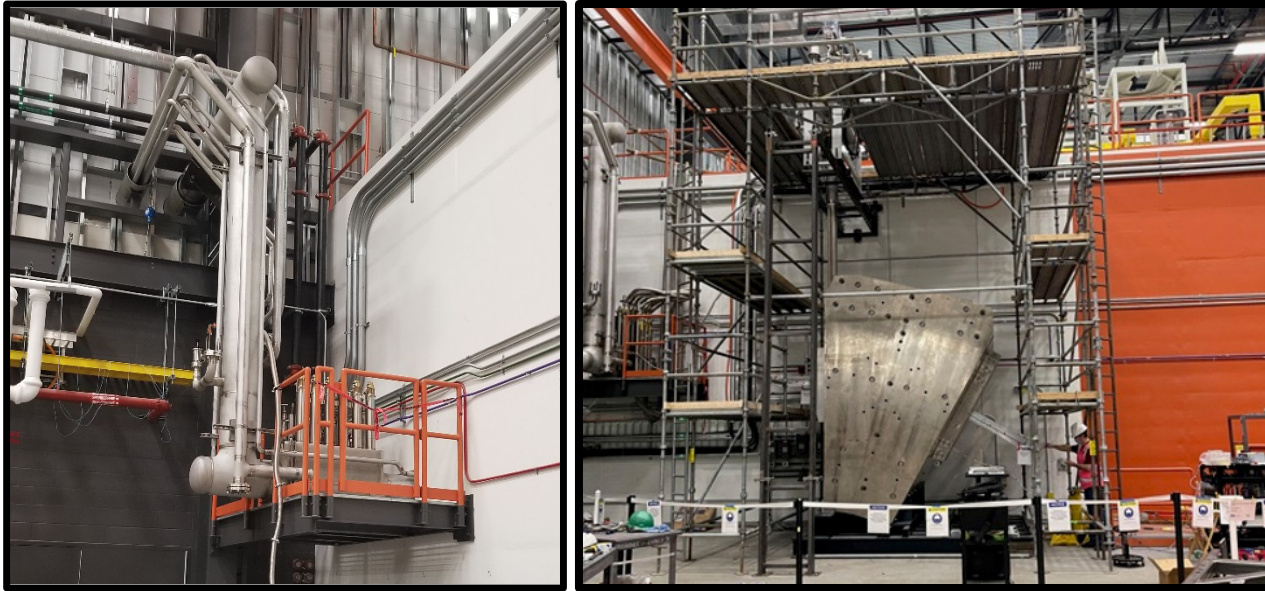
Figure: (left) Magnet Test Station Distribution / Bayonet Box and, (right) SCD1 magnet field mapping ongoing at Magnet Test Station
