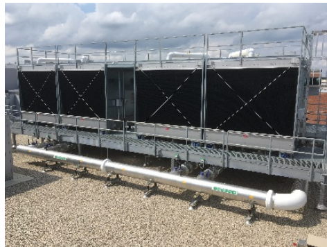
Cooling Tower Loop
